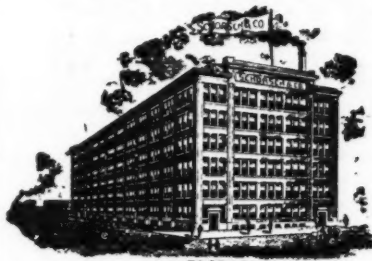
FACTORY 132 ND TO 133 RD ST. & BROOK AVE
